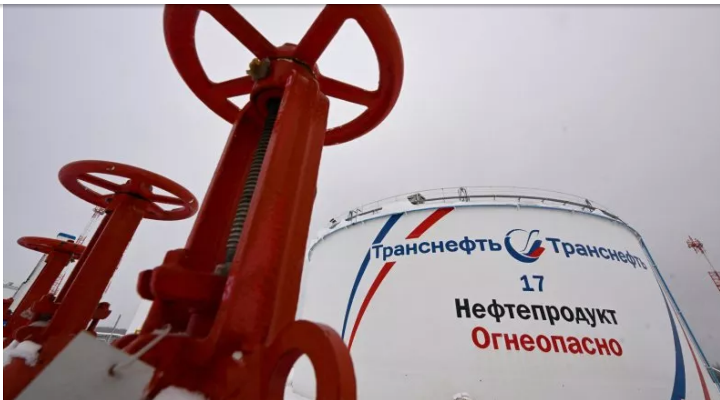
The grounds of a fuel tank farm of Russia's oil pipeline giant Transneft as seen on December 13, 2023. NATALIA KOLESNIKOVA/GETTY IMAGES
